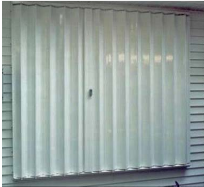
Figure G2-5 Accordion Shutter Closed over window
