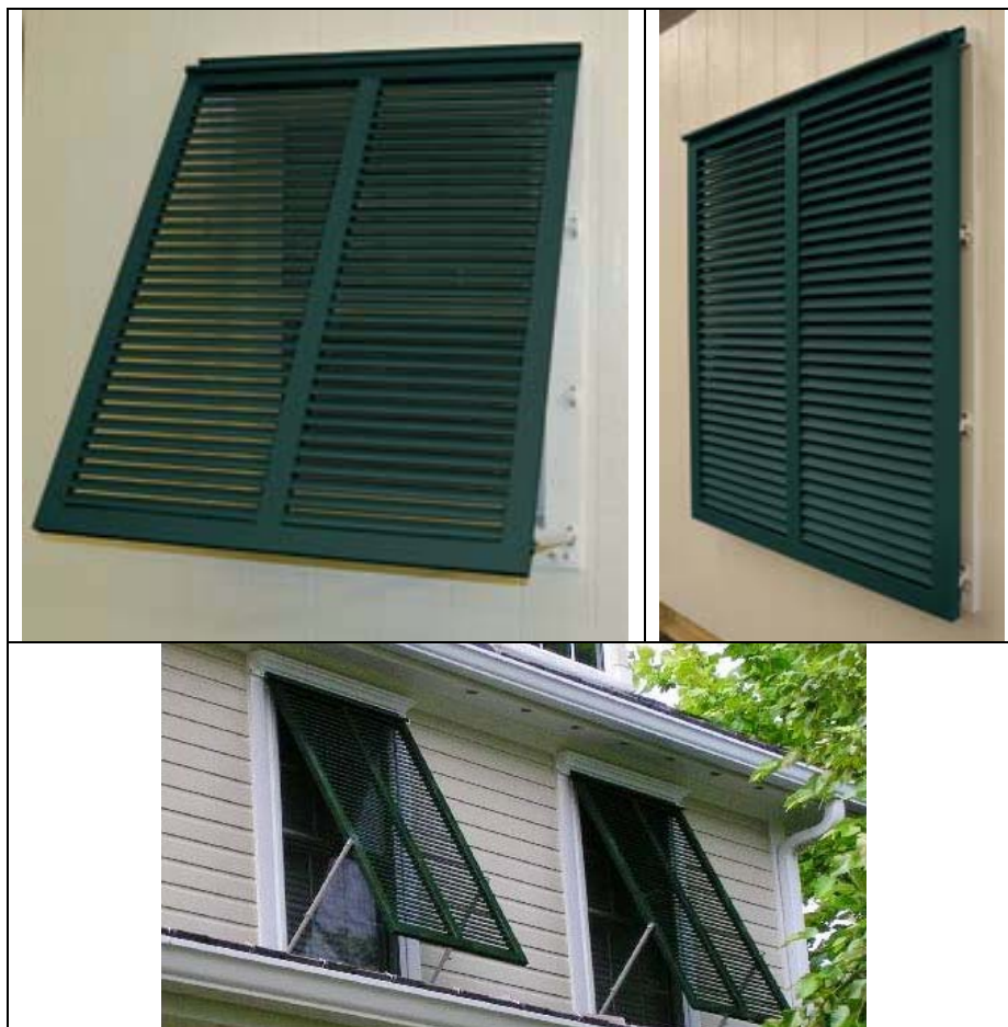
Figure G2-8 Installed Bahama Shutters
