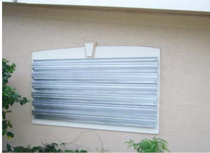
Figure G3-4 Horizontal installed shutters
