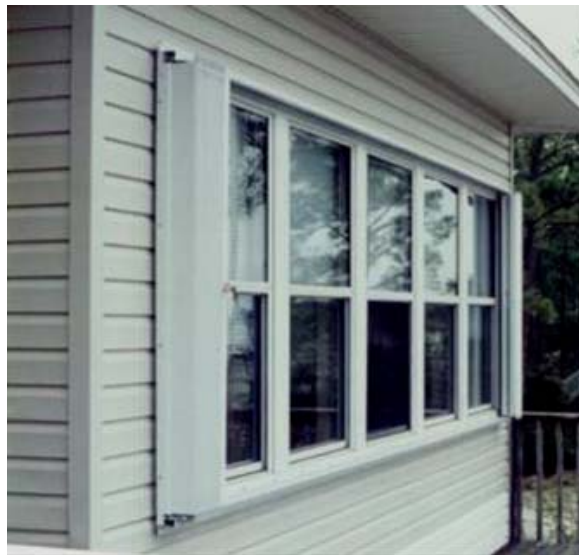
Figure G2-4 Accordion shutter installed
